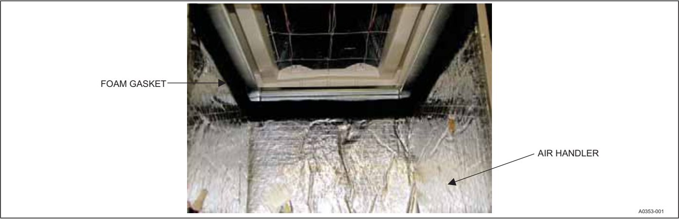
FIGURE 4: Gasket Location
